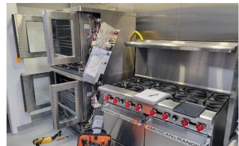
Figure 12: Kitchen maintenance (image credits: freepik.com)
